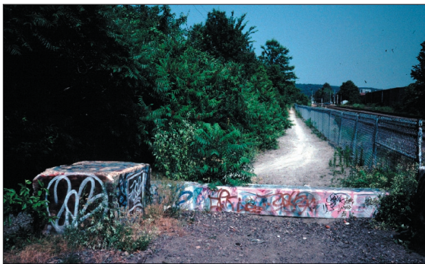
FIGURE 78. The existing, narrow stone dust path parallel to Boston-Maine Railroad tracks
